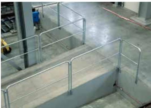
The side brackets are available in right and left-hand versions, and floor brackets are available in single and double versions. These provide a simple, stable fixing and good vertical adjustment options.
